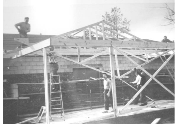
Bill Walsh, Bill Brantley, Tony Petrino, raise rafters for the barbeque cook area (now part of the kitchen.)
