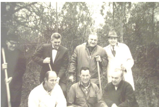
Ready to break ground for the new council home on Spaulding Drive are PGK Paul Hagelston, DGK Bill Brantley, Don Bomba, GK Bill Perkins. In the foreground is Building Chairman Bill Walsh (front left) conferring with Paul Gray and Pope Turner, contractors.
